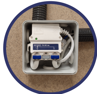
80x 80 mm junction box installation
