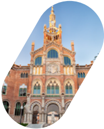
Hospital of Sant Pau Barcelona
